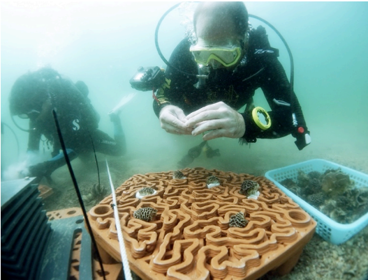
Image 1: A structurally complex foundation for coral attachment with additional elements to aid the removal of sediments from the corals. (Photo Credit: AFCD)
