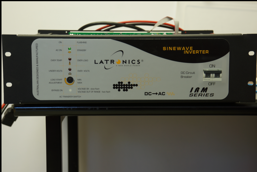
120VDC to 230VAC inverter.
